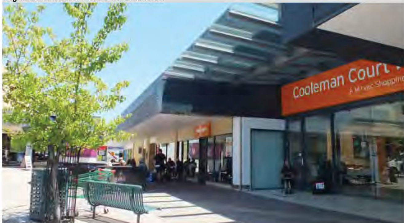
Figure 11: Cooleman Court southern entrance
