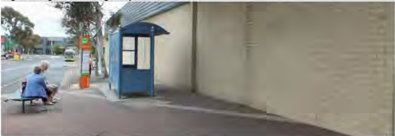
Figure 9: Long blank wall along Brierly Street
