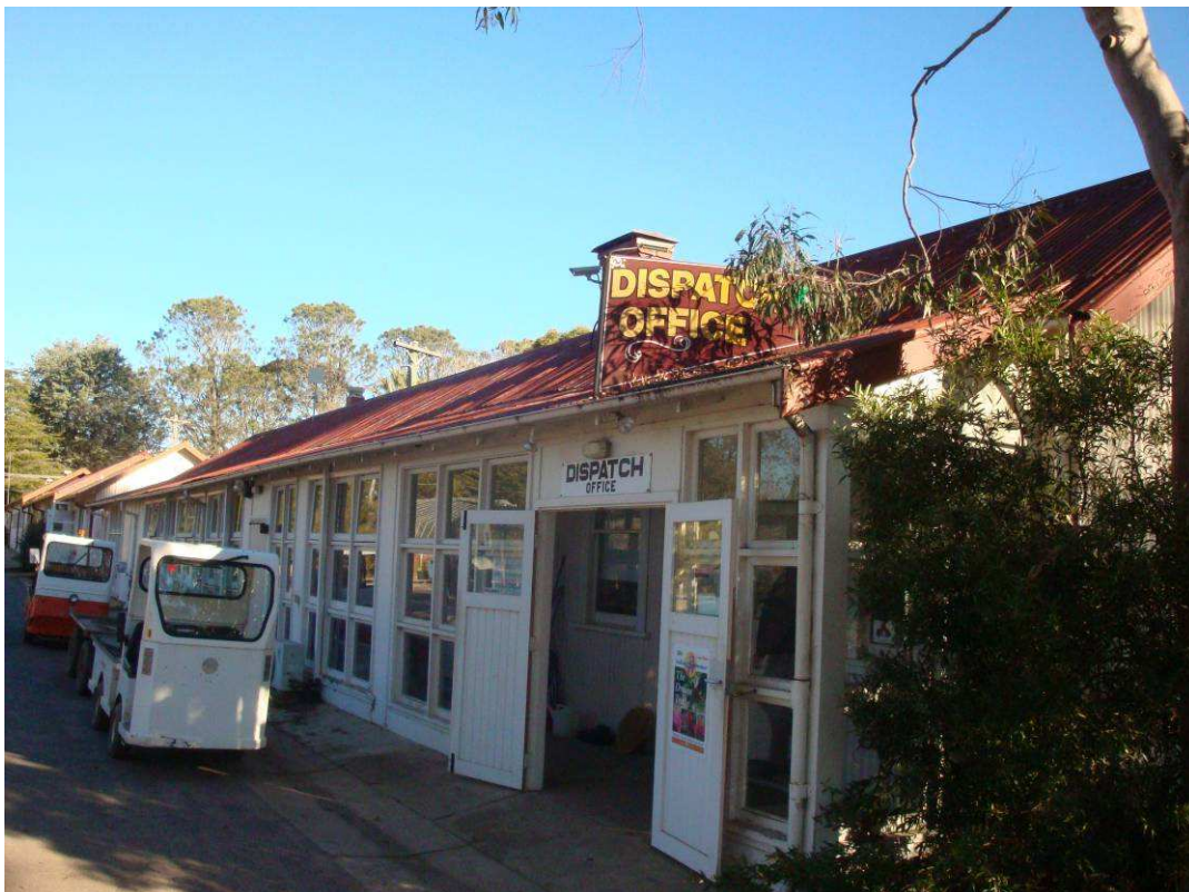
Figure 2.8 Dispatch Office as it is today. (Source: GML 2010.)
