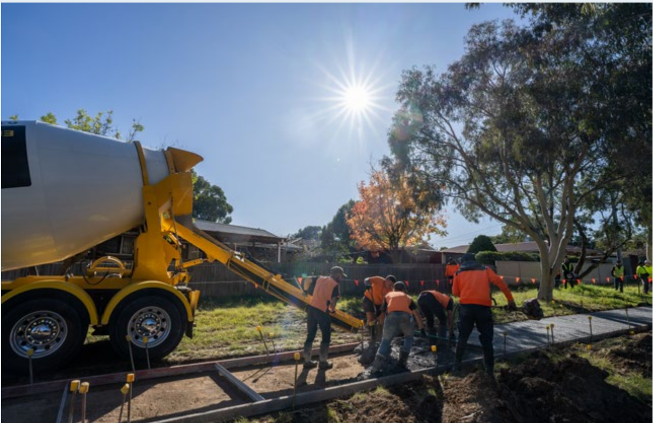
Image depicts concreters and a mixer smoothing over wet concrete to form a community path containing eMesh.
