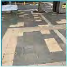
WO38104( AFTER COMPLETION)
