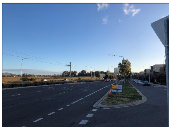
Figure 6. Flemington Road (View North)
