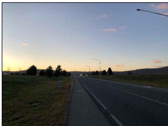
Figure 4. Well Station Drive (View East)
