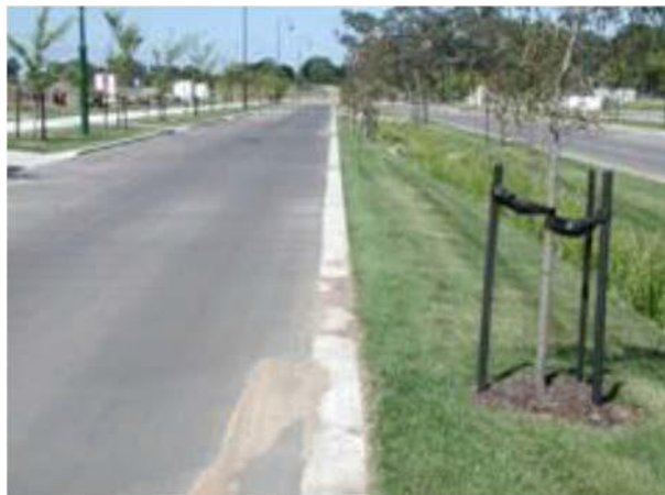
Figure 8- 34 Flush kerb without setdown, showing sediment accumulation on road
