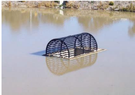
Figure 8- 24 Typical primary outlet domed cover
