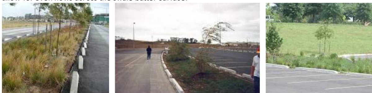
Figure 8- 33 Bioretention swale kerb treatments
