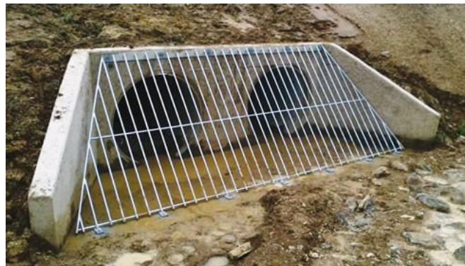
Figure 8- 9 Typical culvert inlet protection grate
