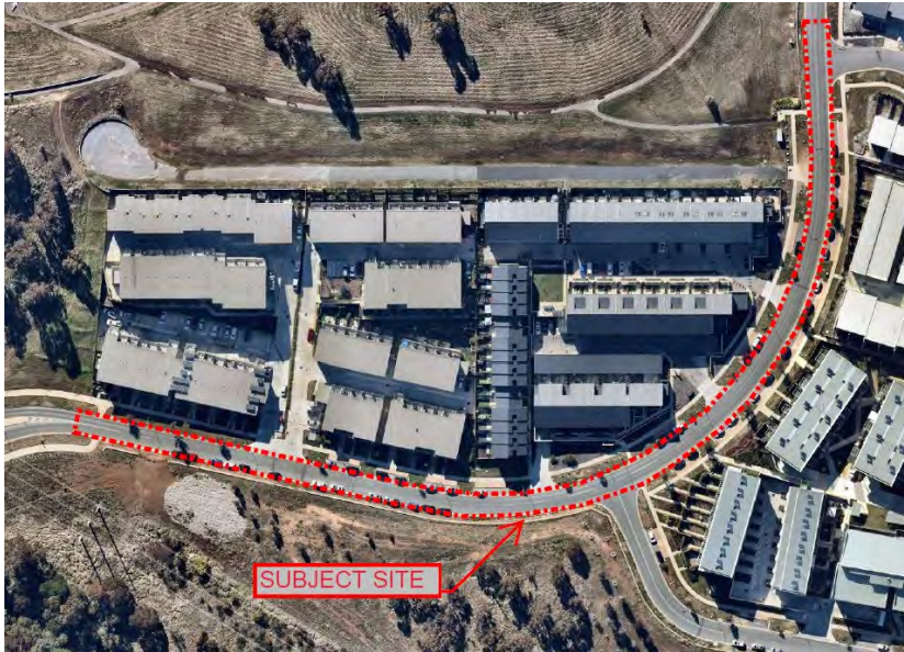
Figure 2-4 Section 21 – Parking survey area
