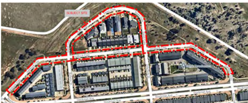
Figure 2-5 Section 45 – Parking survey area
