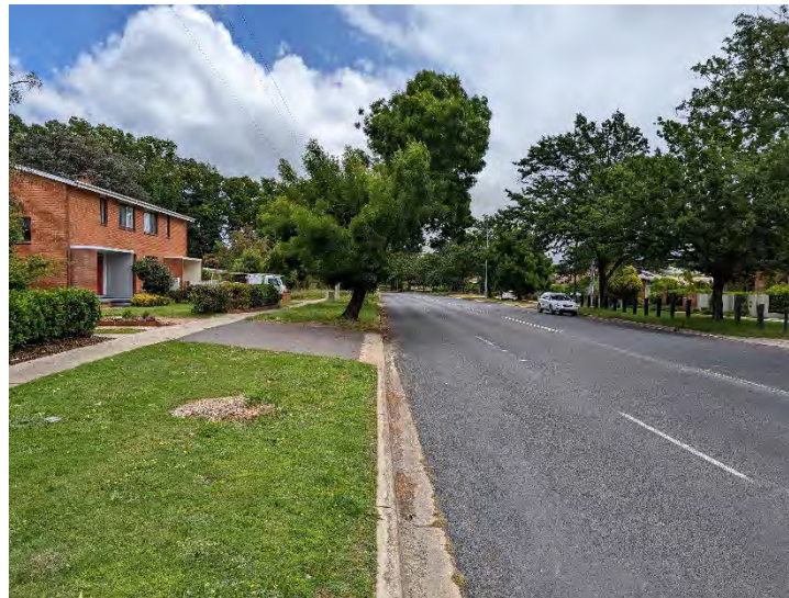
Photo 6-15 Majura Av (westbound view west of the intersection with Cowper St)
