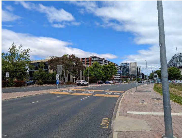
Photo 6-27 Cooyong St (southbound view south of the intersection with Torrens St)
