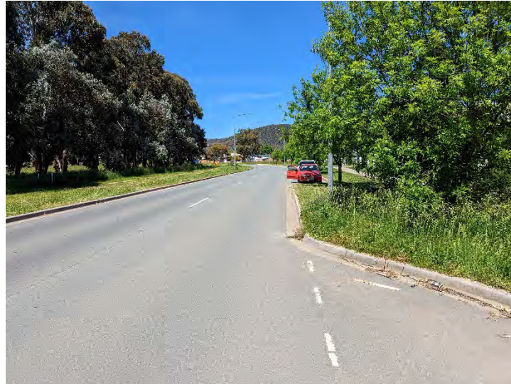
Photo 6-2 Aspinall St (eastbound view west of the intersection with Negus Cr)
