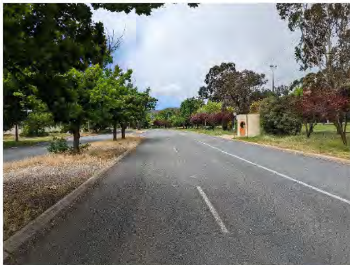
Photo 6-9 Antill St (eastbound view west of the intersection with Cadell St)
