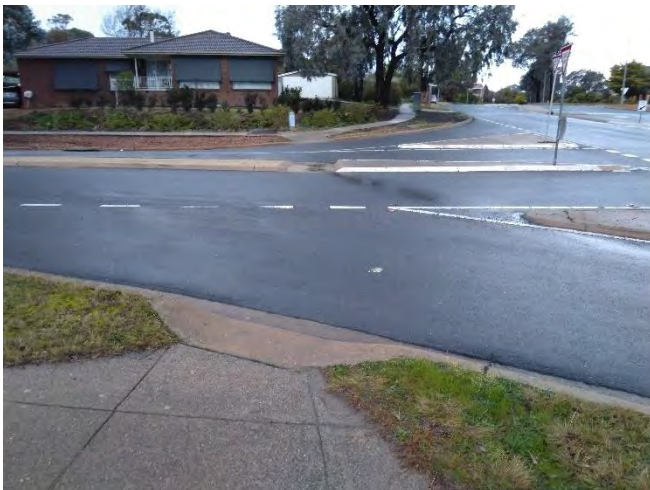
Figure 14 Pedestrian Paths and Kerb Ramps – Marconi Crescent
