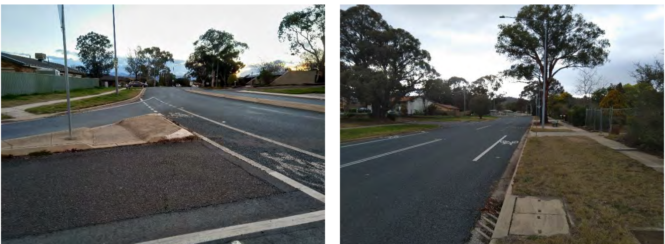
Figure 8 Discontinuous On-Road Bicycle Lanes
