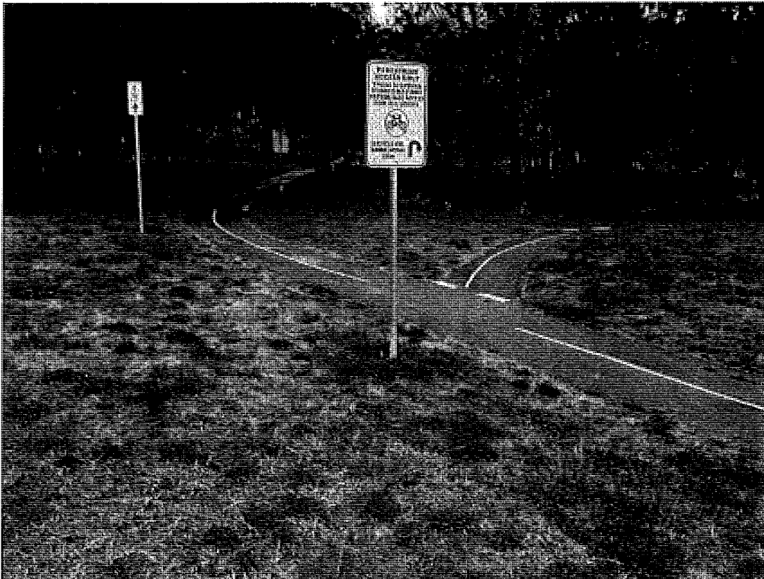
Figure 5-2 Photo 13: Centreline cycleway line markings on approach path to stepping stones
