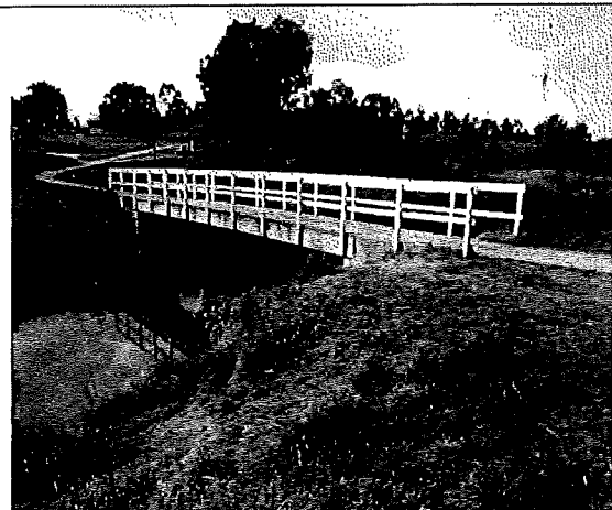
Figure 2-8 Photo 7: Macrossan Crescent footbridge
