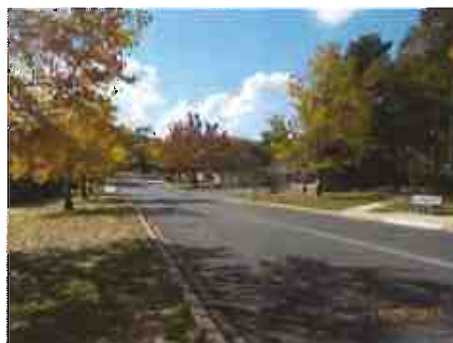
Figure 4: 114m South on Blamey Crescent
