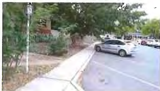
View east at entry through along northern façade
