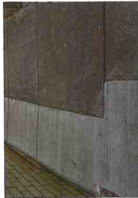
2 Tired concrete paving - mixed concrete finished and colours
