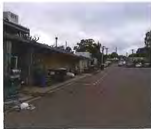
Cracked and tired pavements
