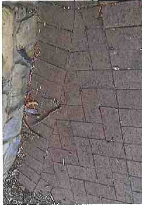
3 Old unit paving
