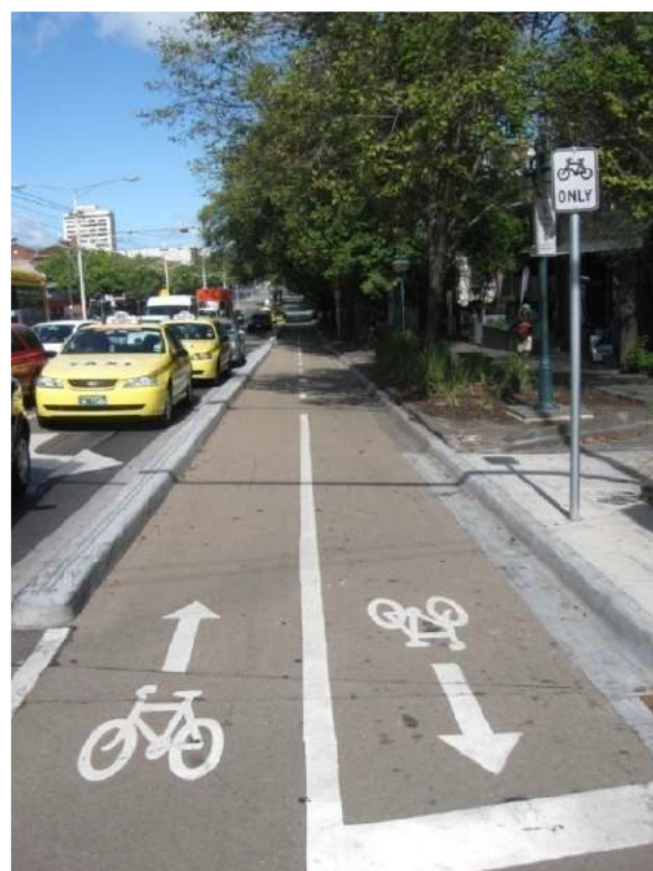
Figure 4-3 Bi-directional path in carriageway, St Kilda, Melbourne (Complete Streets Guidelines for Urban Street Design)
