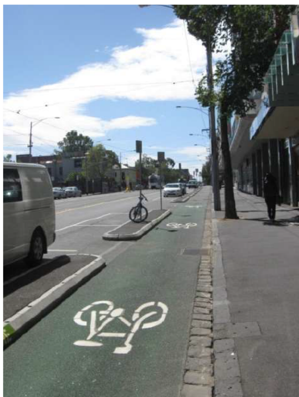
Figure 4-2 Separated bicycle lane, Swanson Street, Melbourne (Complete Streets Guidelines for Urban Street Design)
