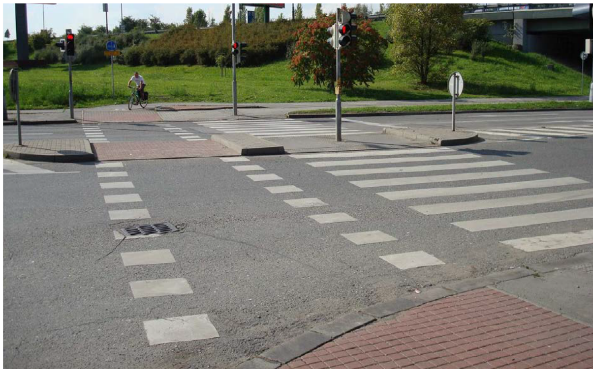
Figure 4-8 User separation through signalised intersection
