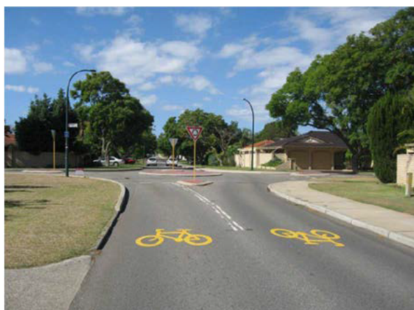
Figure 4-6 Macrae Road and Train Street, Perth 9
