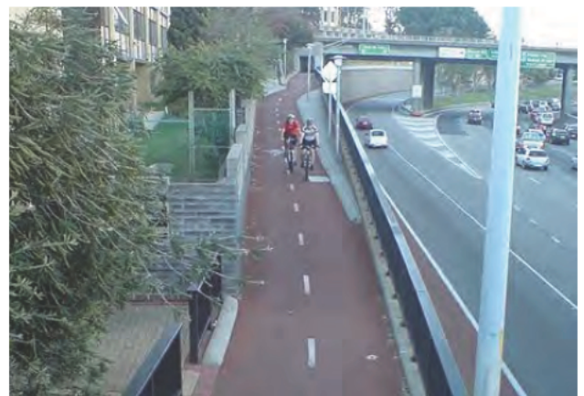
Shared path adjacent freeway 6
