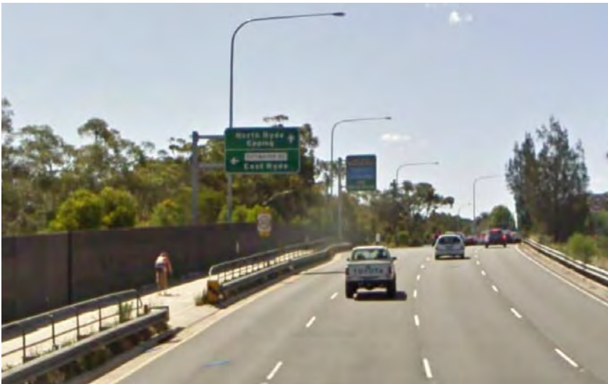
Epping Road Sydney NSW. Cycleway separated from roadway by crash barrier.
