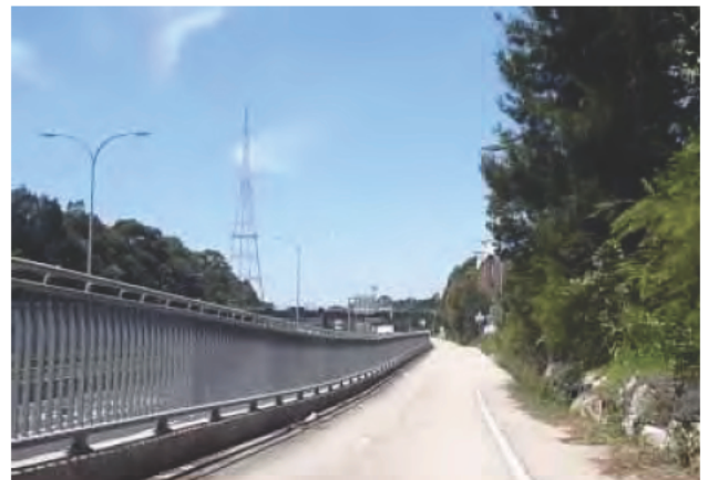
Separated Cycleways: Vertical barrier
