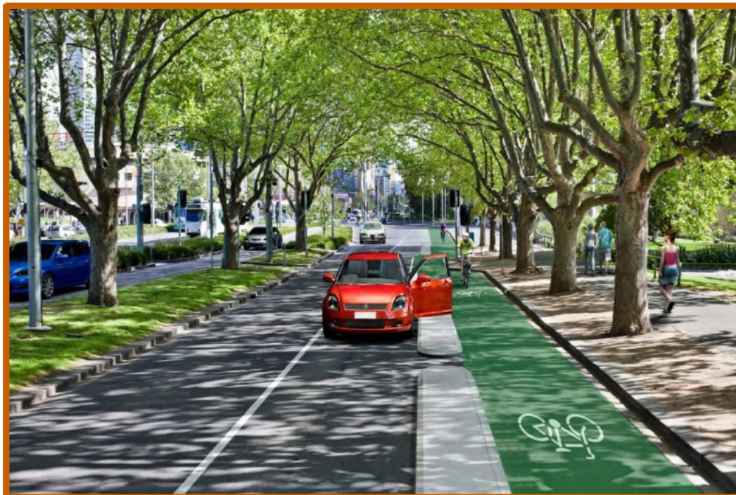
Figure 3: Example of an on-road segregated lane concept in Melbourne that provides protection from traffic and casual surveillance from neighbouring uses and passing traffic
