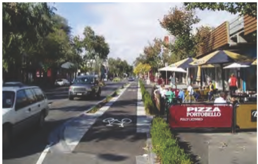
One-way separated cycleway - Melbourne, Victoria
