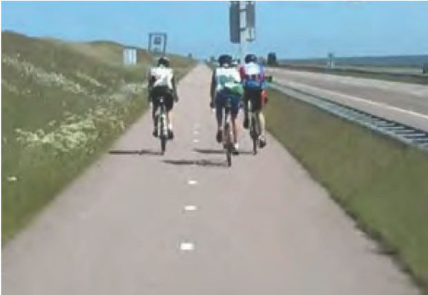
Separation from road with grass verge 1
