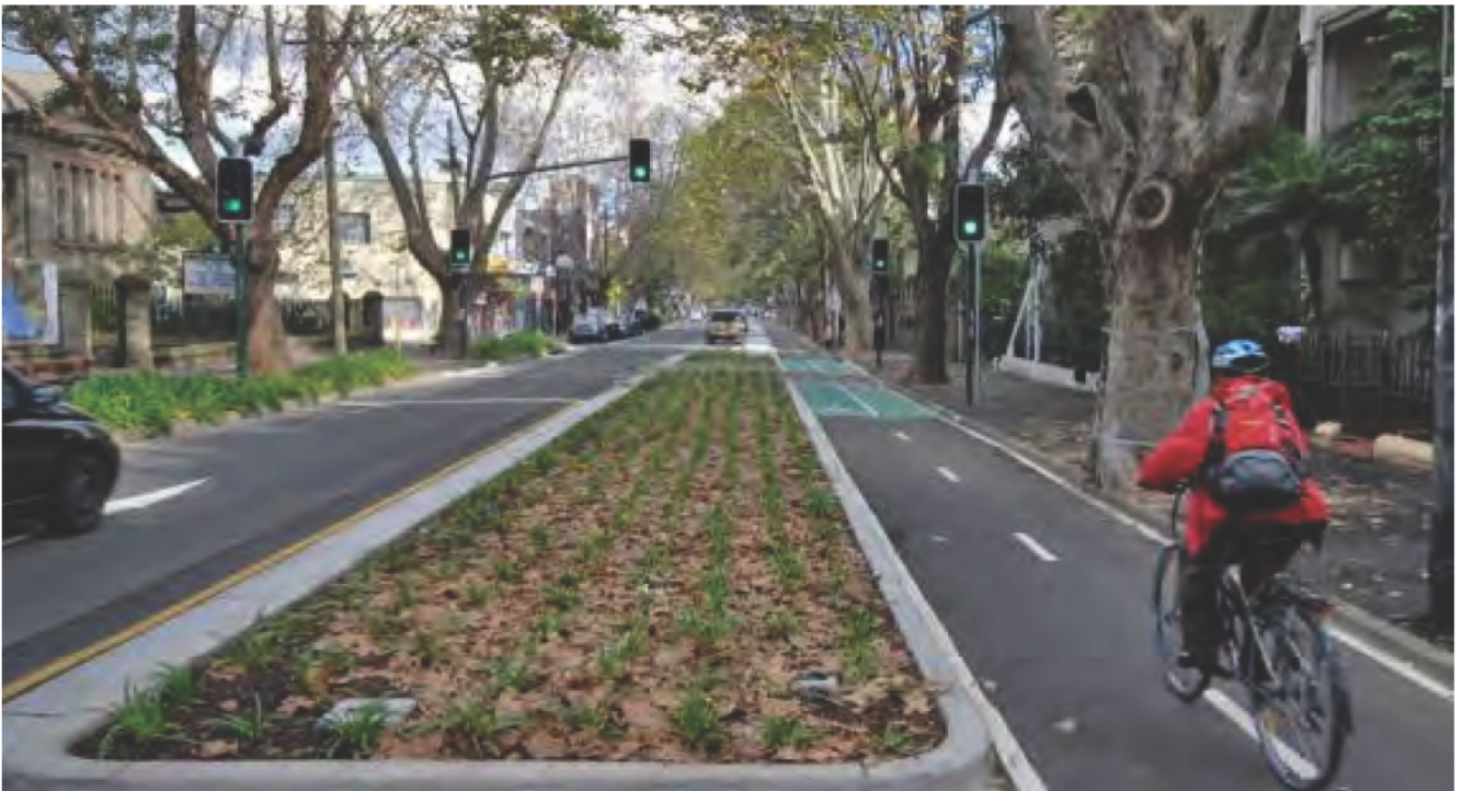
Bi-Directional Cycleway with planted median island
