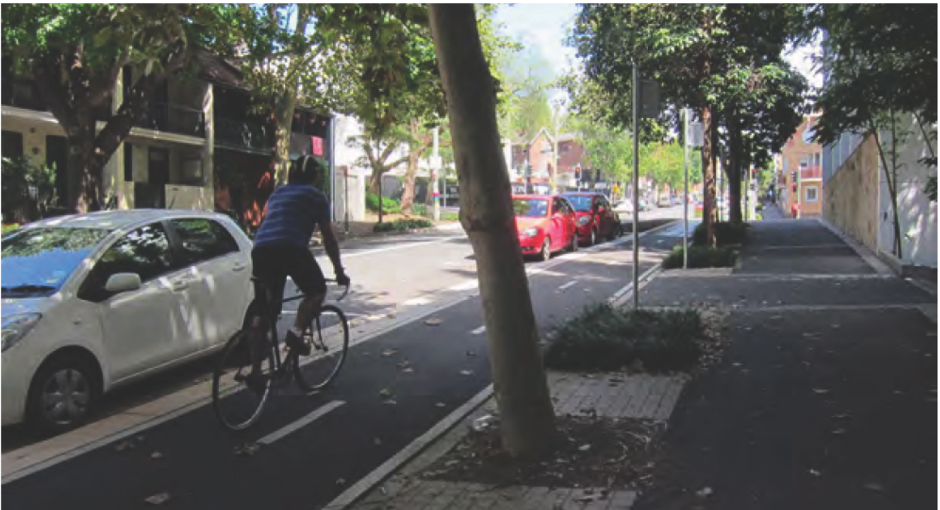
Bi-Directional Cycleway at grade with footpath
