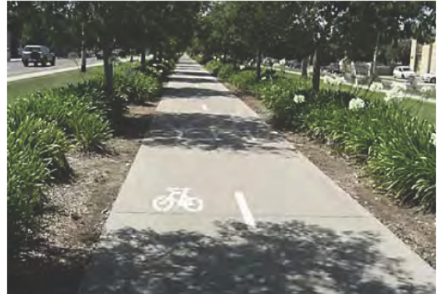
Shared path in central median with planting either side 2
