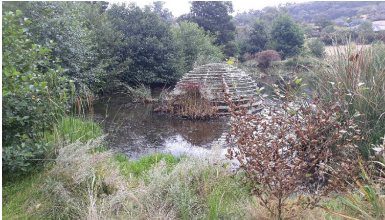
Figure 3 – Overflow inlet structure
