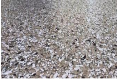
Granulated epoxy chip trowelled grout floor finish to internal areas.
