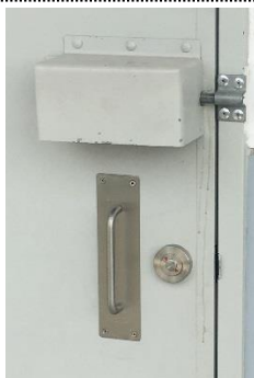
External door with slide bolt / pad bolts and padlocks in security shroud. Door pull handle and Privacy latch.
