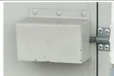
External door with slide bolt / pad bolts and padlocks in security shroud.
