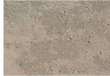
Non-slip concrete floor finish to external areas.
