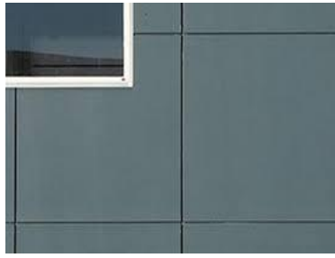
Pre-finished compressed fibre cement – panelized wall lining.
