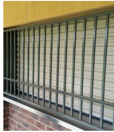
Food Servery roller shutter, with security gates, pad bolts and padlocks.
