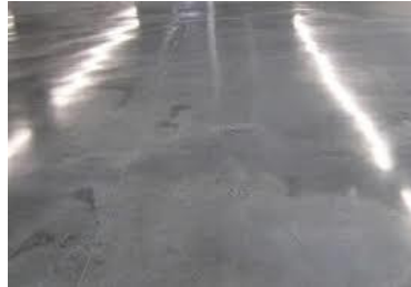
Sealed concrete floor finish to internal areas.
