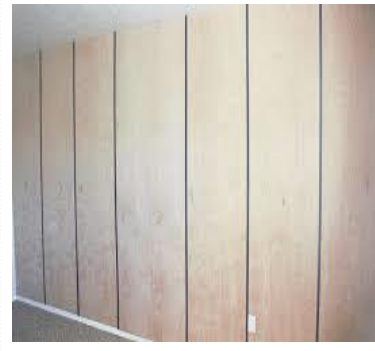
Smooth plywood wall lining / finish.
