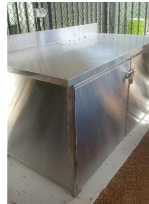
Lockable stainless steel BBQ storage bench and cupboard. Note ant-bed gravel to front in lieu of concrete and waterproof GPO behind.
