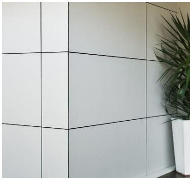
Compressed fibre cement – panelized wall lining / finish.
