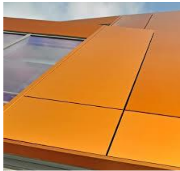
Pre-finished compressed fibre cement – panelized wall lining.
