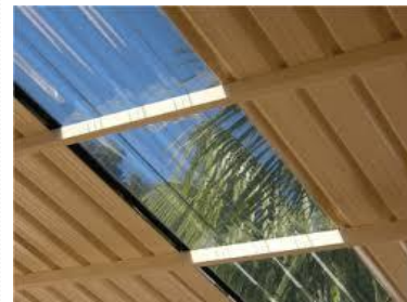
Translucent (frosted) roof panels with security bars / grilles below.
