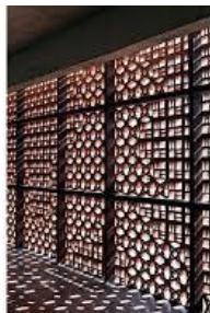
Perforated metal screens that do not provide privacy – Not to be Used.
