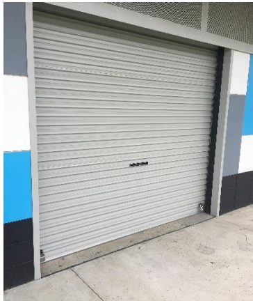
Roller shutter, with security slats and bottom rail with multiple locking pad bolts and padlocks.
