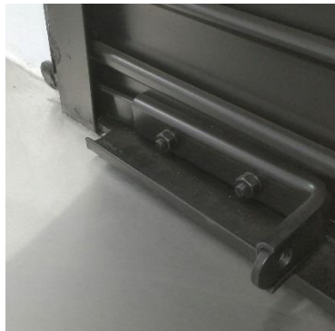
Roller shutter door with slide-bolt, and base security angle slat.
