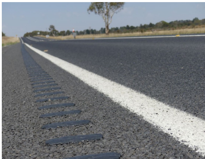
Figure 3: Example of black ATLM installed on edge lines
