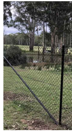
FE1 1.8M HIGH CHAIN LINK FENCE
