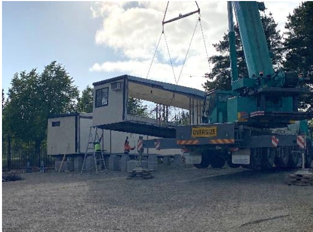
Image 1 Installation of demountable buildings at Curtin works depot
