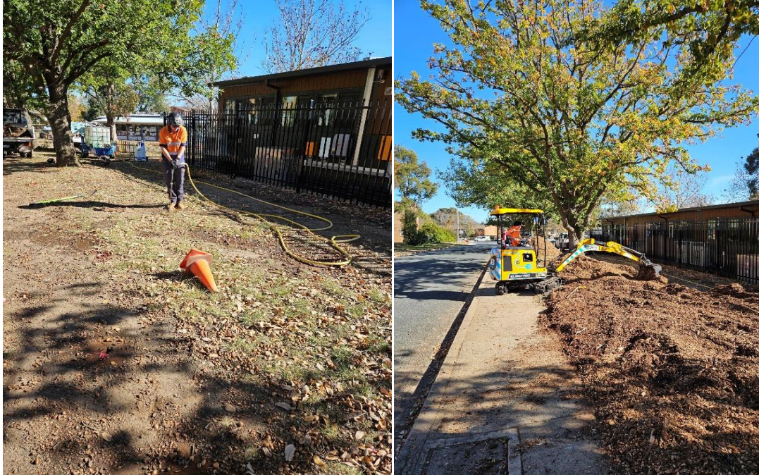
Image 4 Treatment of compacted soil surrounding the subject street trees
