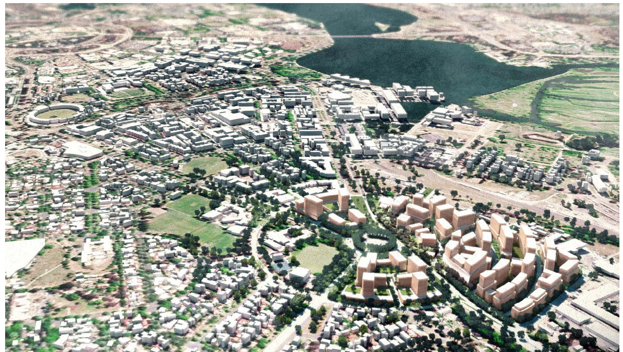
Figure 1. Aerial view of potential development in the Hume Circle Precinct (OCULUS, Warren & Mahoney)
