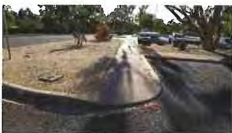
Non-compliant kerb ramps
