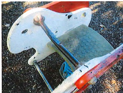
Photo taken: 23/05/2016 Bent hand support, monitor.
