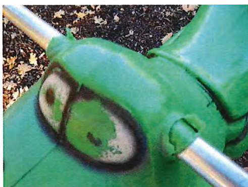
Photo taken: 25/05/2017 Plastic peeling. Monitor.
