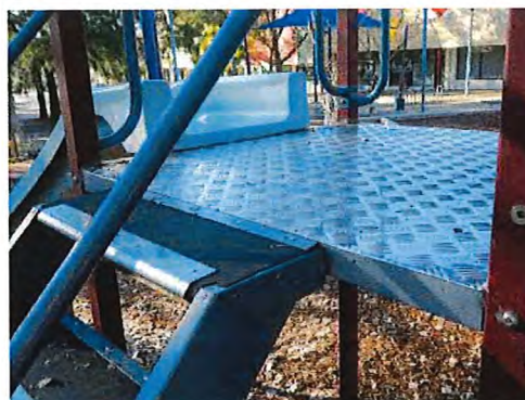
Photo taken: 25/05/2017 Slide deck covered with aluminium sheeting.
