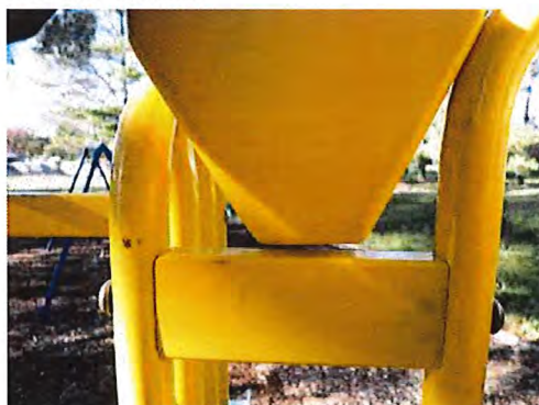
Photo taken: 13/05/2010 Neck probe just not touching the bottom
