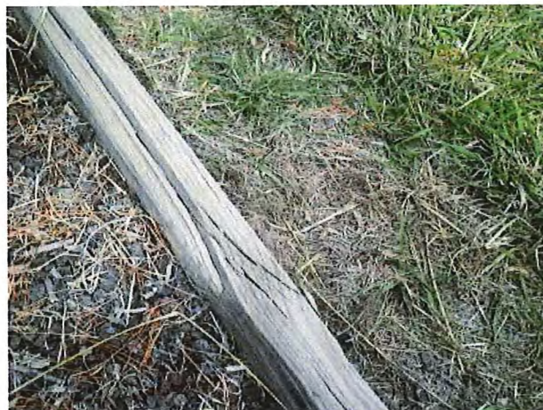
Photo taken: 03/05/2011 Some sections of timber edging exhibit splitting. Monitor.
