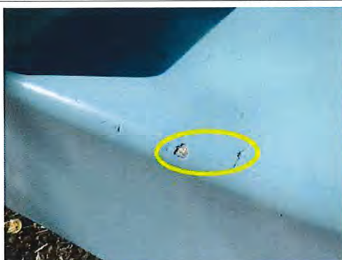
Photo taken: 23/05/2016 Small chips in slide, monitor.
