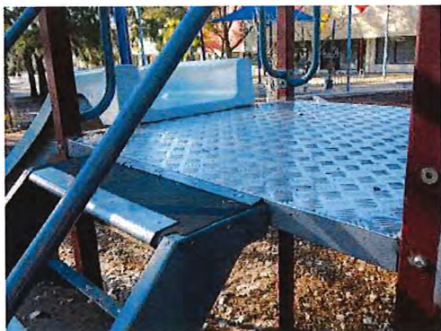
Photo taken: 25/05/2017 Slide deck covered with aluminium sheeting.
