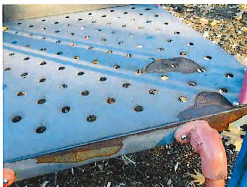
Photo taken: 25/05/2017 Deck coat peeling. Monitor.
