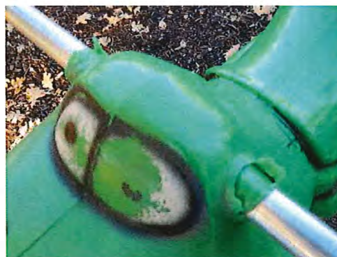
Photo taken: 25/05/2017 Plastic peeling with sharp edges. Monitor.
