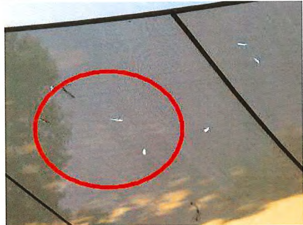
Photo taken: 18/04/2018 Holes in shade cloth. Monitor.
