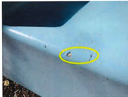
Photo taken: 23/05/2016 Small chips in slide, monitor.
