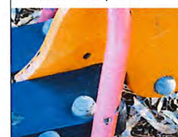
25/05/2017: Missing bolt in tail.
