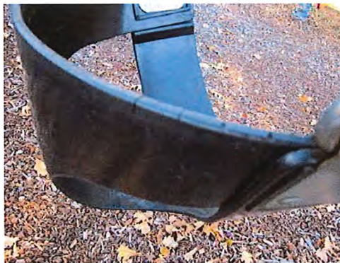
Photo taken: 01/05/2012 Cuts along top edge of toddler seat. Monitor.
