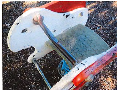
Photo taken: 23/05/2016 Bent hand support, monitor.
