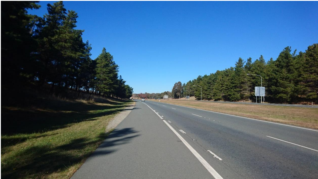
Photo 2-1 Barton Highway (southbound view south of the roundabout with William Slim Drive/ Gundaroo Drive)
