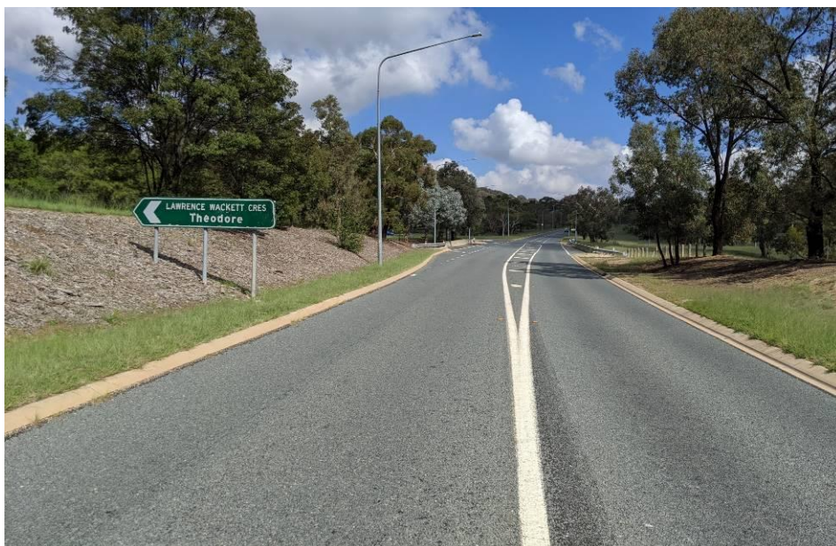
Photo 2-2 Tharwa Drive (westbound view east of the intersection with Lawrence Wackett Crescent)
