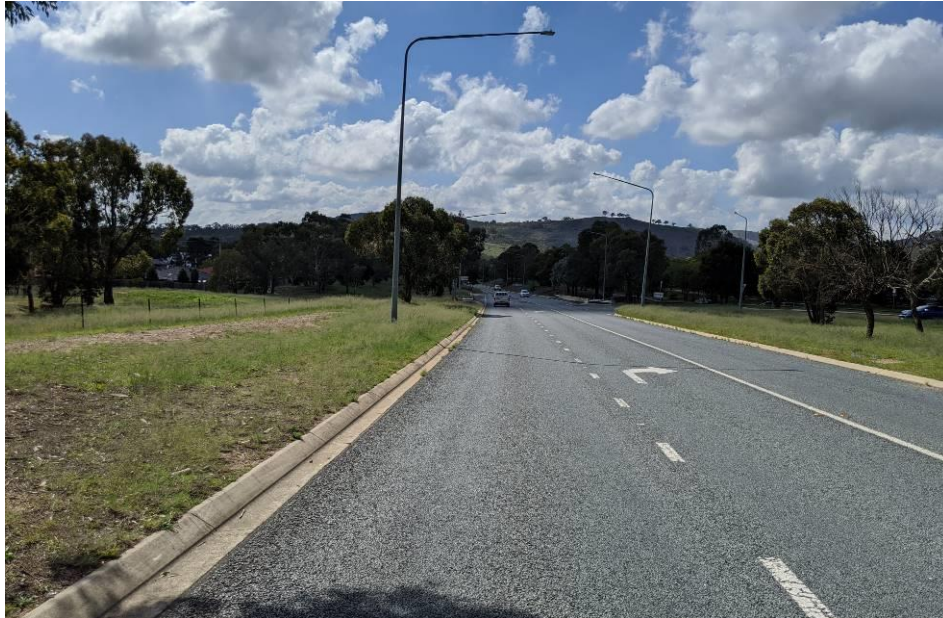
Photo 2-1 Tharwa Drive (eastbound view west of the intersection with Lawrence Wackett Crescent)
