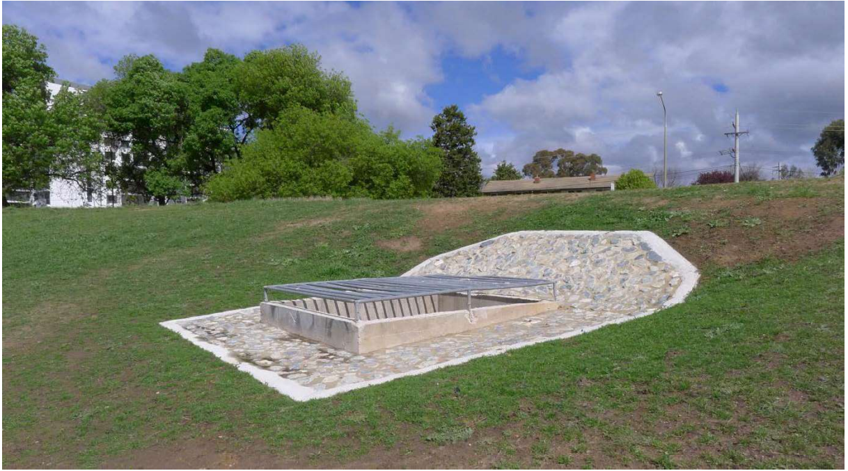
Figure 2-3 Southwell Park basin high level outlet pit
