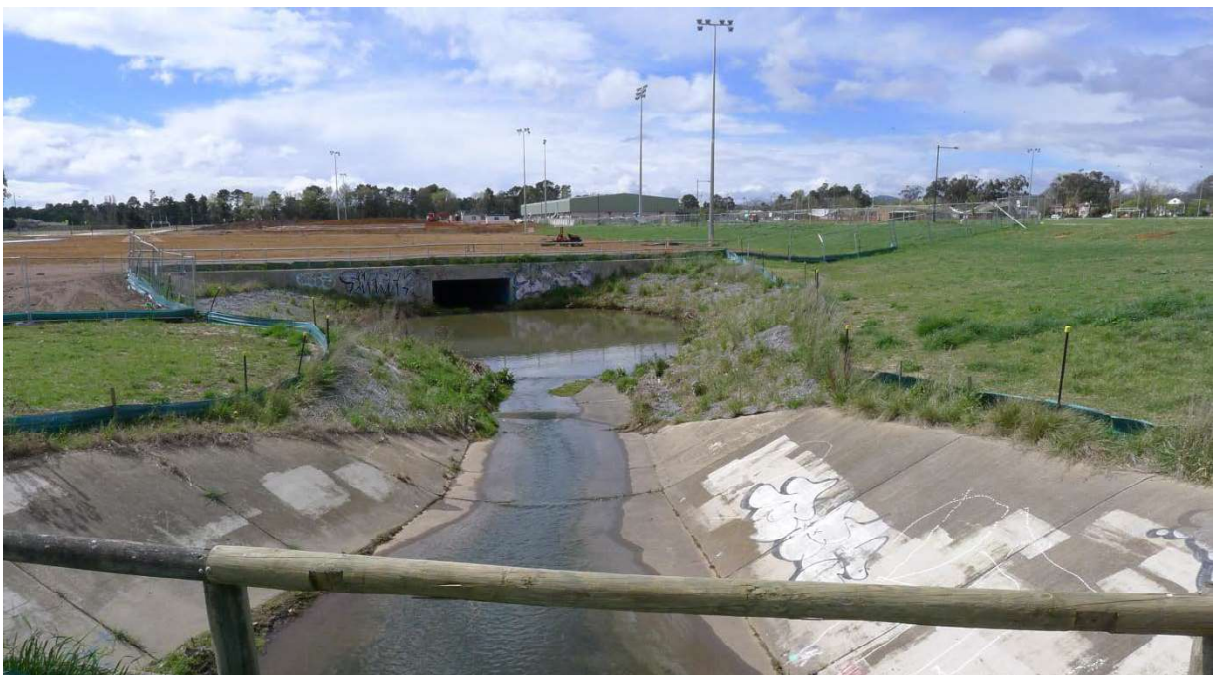
Figure 2-4 Southwell Park inlet culvert and gauge location (in centre)
