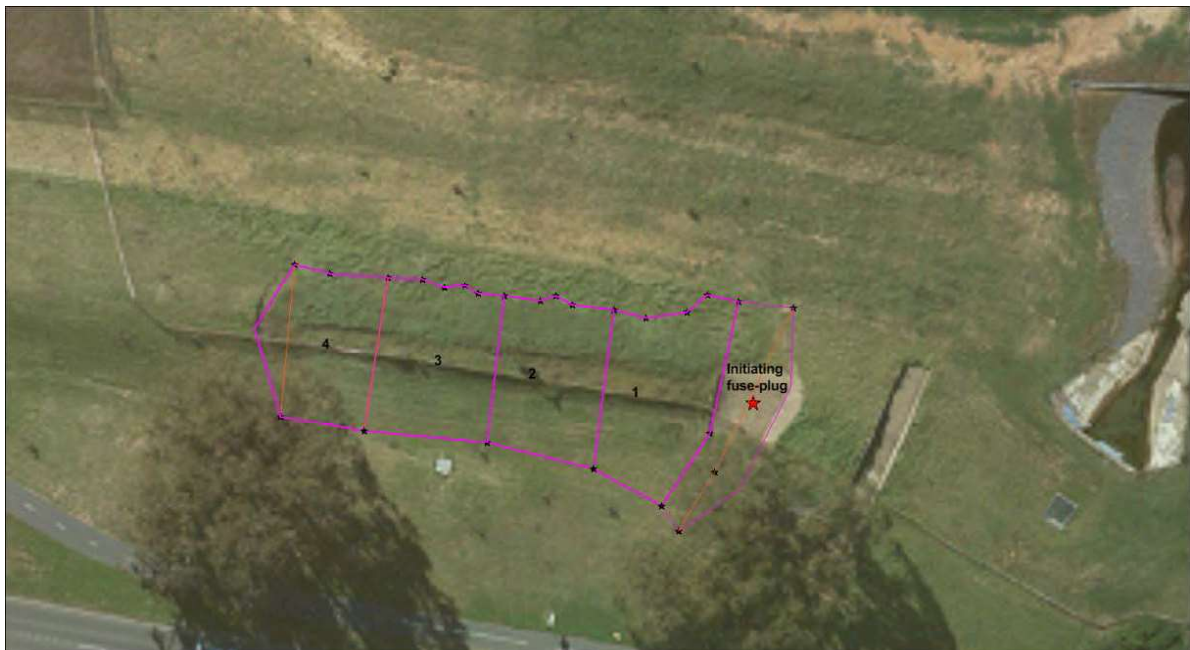
Figure 5-3 Southwell Park fuse-plug spillway
