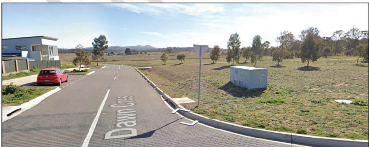
Figure 3-6 Indented car parking and existing verge Dawn Crescent
