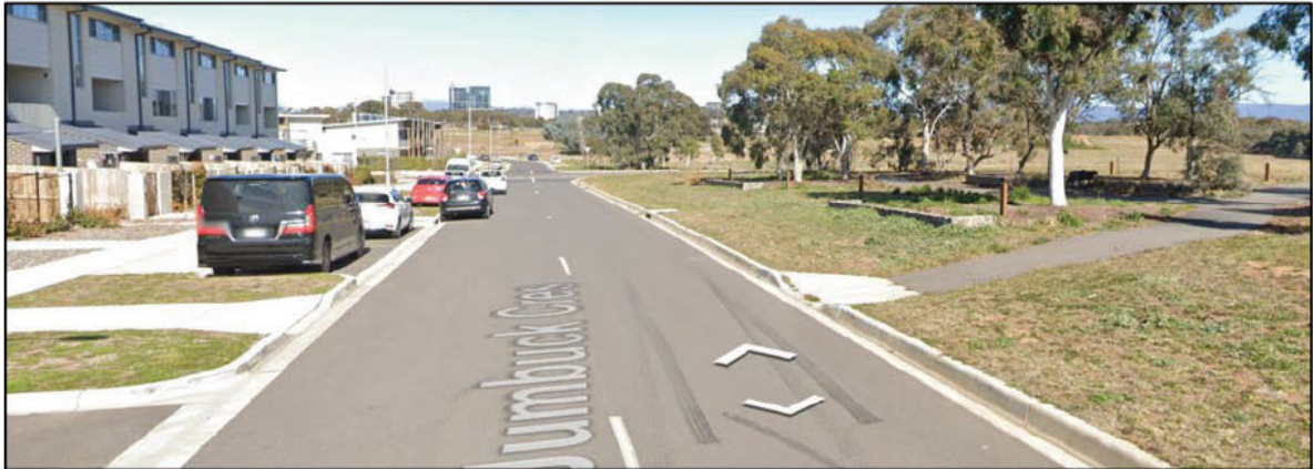
Figure 3-10 Jumbuck Crescent existing road details showing existing indented car parking
