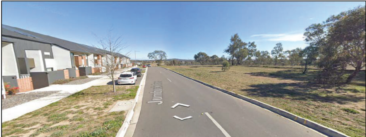
Figure 3-14 Jumbuck Crescent – Section 3 - existing road details
