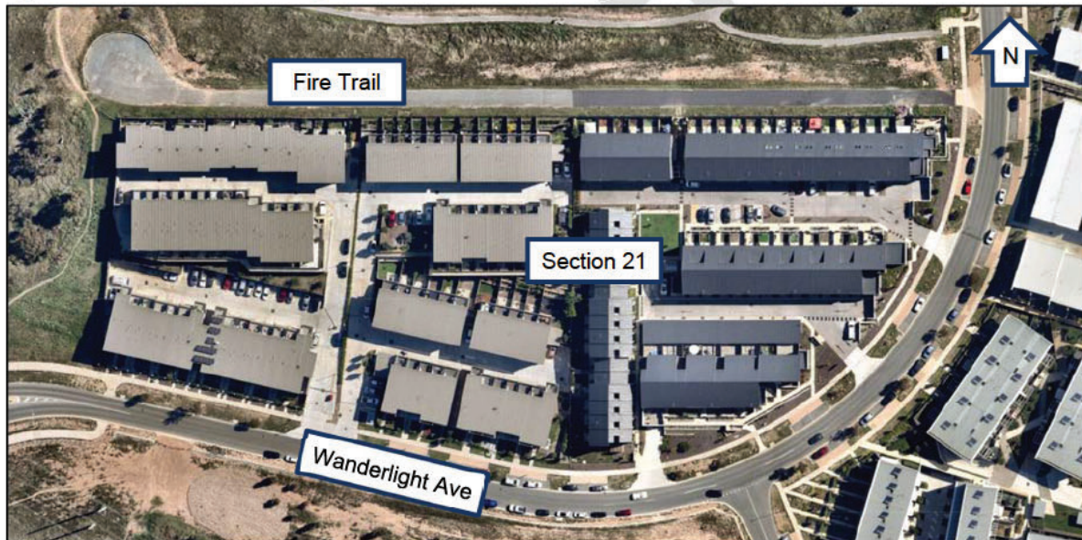
Figure 3-1 Aerial view of Wanderlight Avenue and the fire access road
