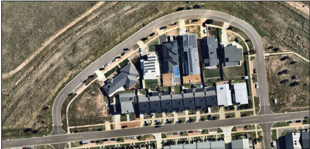
Figure 3-5 Aerial view of Dawn Crescent
