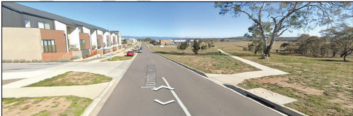
Figure 3-13 Jumbuck Crescent – Section 2 - existing road details
