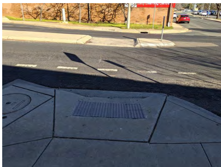
Photo 4 – Crossing Location 2, westbound view from the eastern side of Bowman Street
