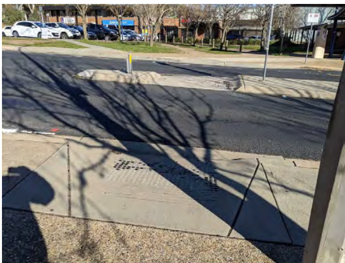
Photo 6 – Crossing Location 3, westbound view from the eastern side of Bowman Street
