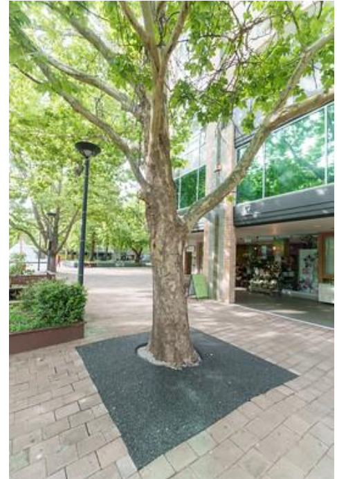
Image 11 City Walk permeable paving repair
