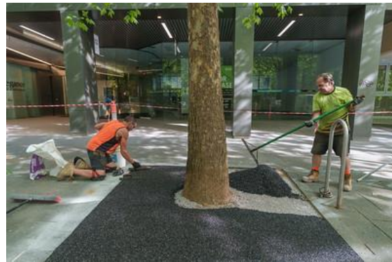
Image 12 Petrie Plaza, City before and after permeable paving installation
