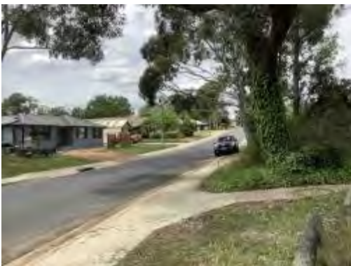
Photo 1 – Pickworth St, large tree obscures sight distance
