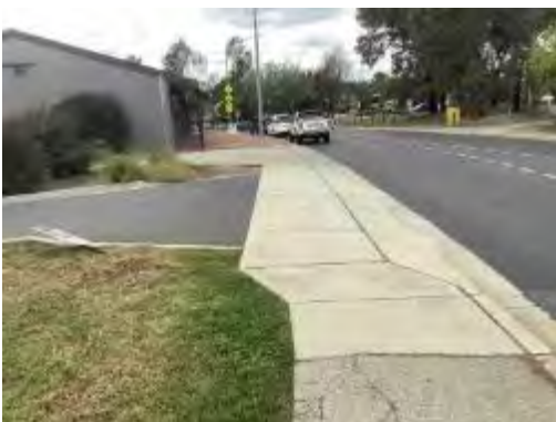
Photo 5 – Driveways across verge on Luke Street
