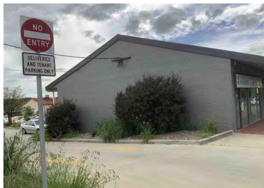
Photo 8 – Entry to eastern carpark is for delivery access and tenant parking only
