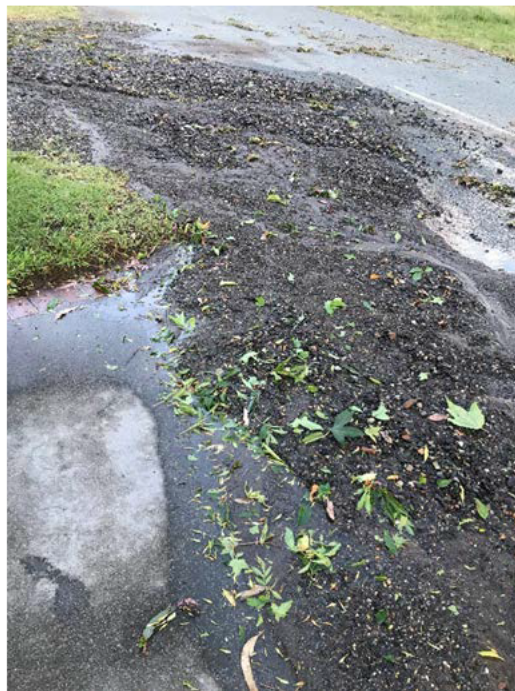
Gravel washed onto Gladstone Street
