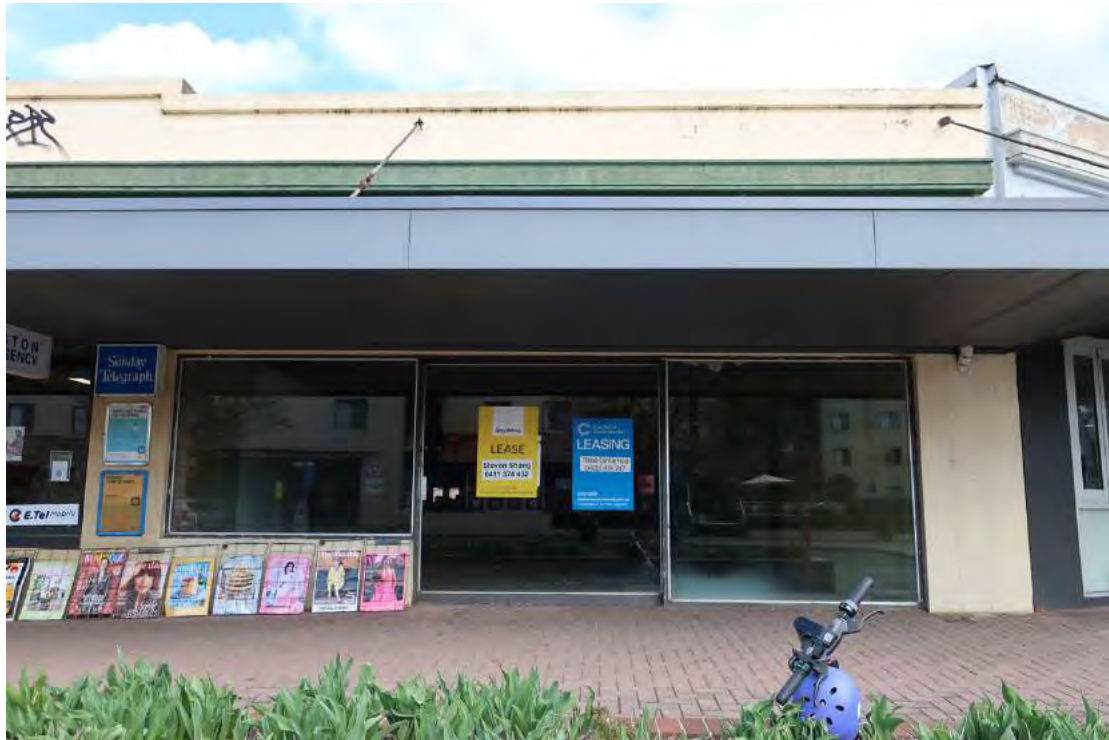
Shopfront to subject tenancy with later aluminium framed windows and door.
