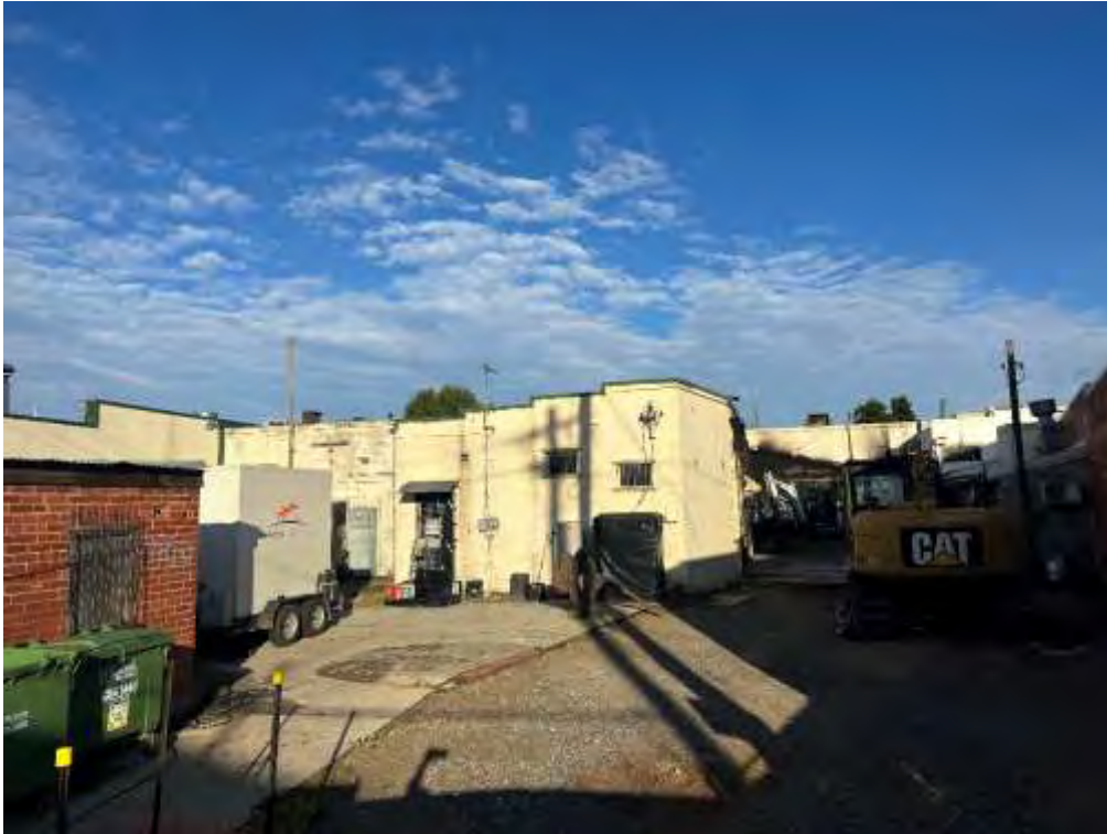
Image 11. View of the rear of the property
