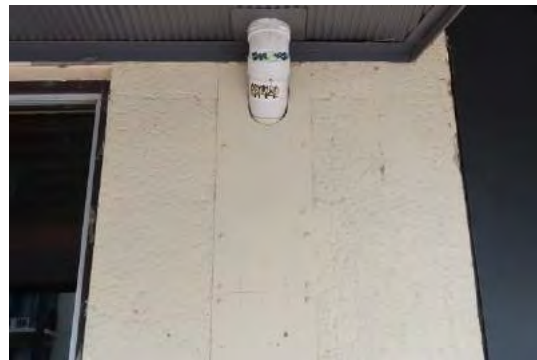
Textured render applied to wall with cover sheet for PVC downpipe
