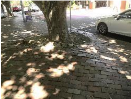
Manuka shopping centre - New Root Pave product has been contoured over existing structural tree roots and trip hazards have been eliminated.
