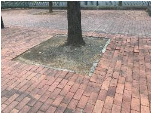
Glebe Park - Root Pave product finished level with surrounding pavement. Root Pave product has a high porosity rate, is flexible and trafficable.
