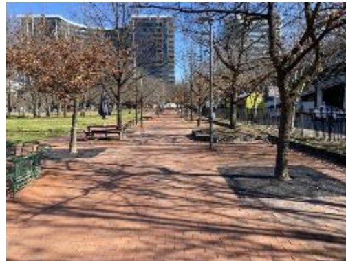
Glebe Park - Root Pave product finished level with surrounding pavement. Root Pave product has a high porosity rate, is flexible and trafficable.
