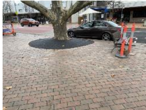
Manuka shopping centre - New Root Pave product has been contoured over existing structural tree roots and trip hazards have been eliminated.
