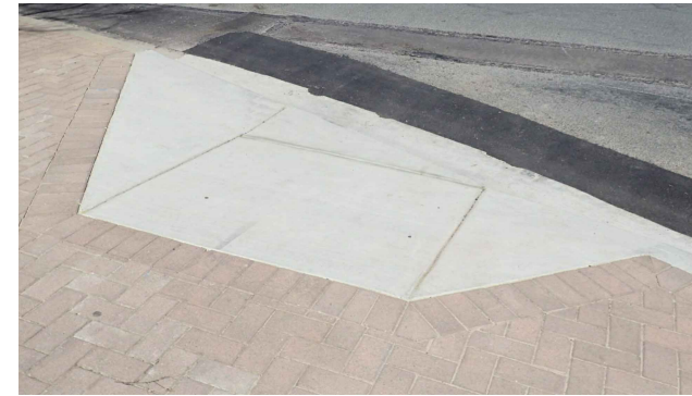
EXAMPLE OF INNER URBAN KERB RAMP
