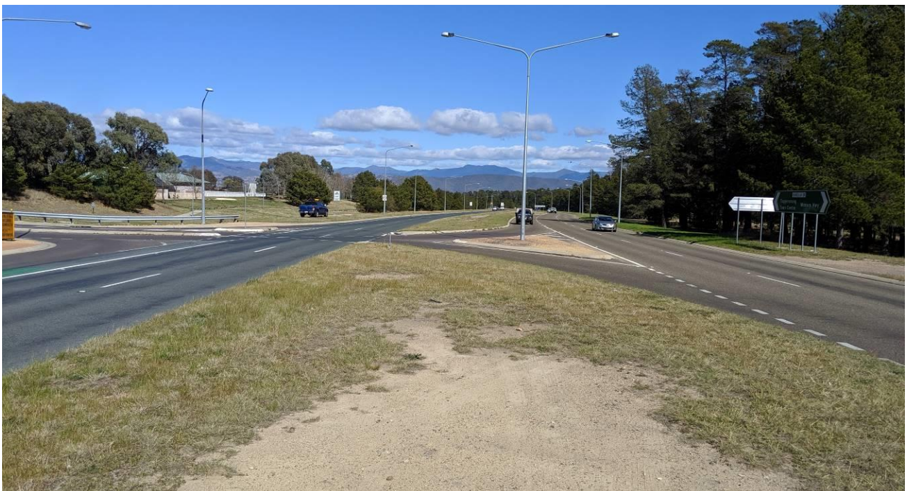
Photo 2-2 Isabella Drive (westbound view east of the intersection with Benham Street)
