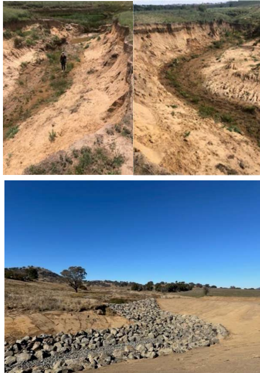
Figure 2. Top – the eroding creekline on a landholders property prior to remediation works. Bottom – the creekline after remediation works.
