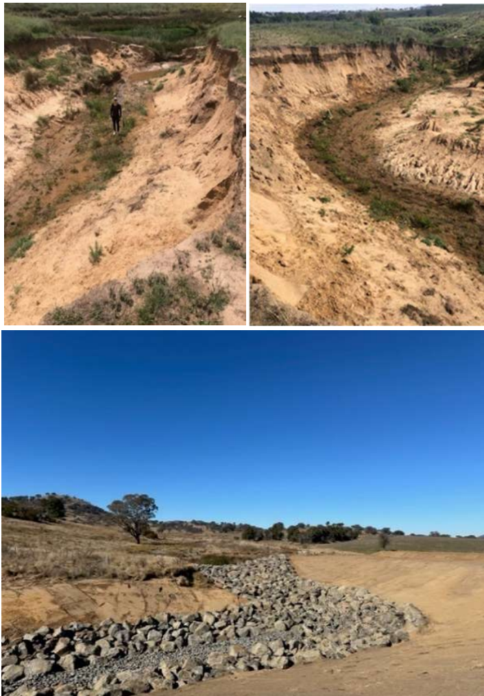
Figure 2. Top - the eroding creek line on a leaseholder's property prior to remediation works. Bottom - the creek line after remediation works.
