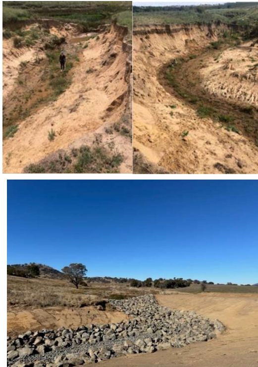
Figure 3. Top – the eroding creek line on a leaseholder's property prior to remediation works. Bottom – the creek line after remediation works.
