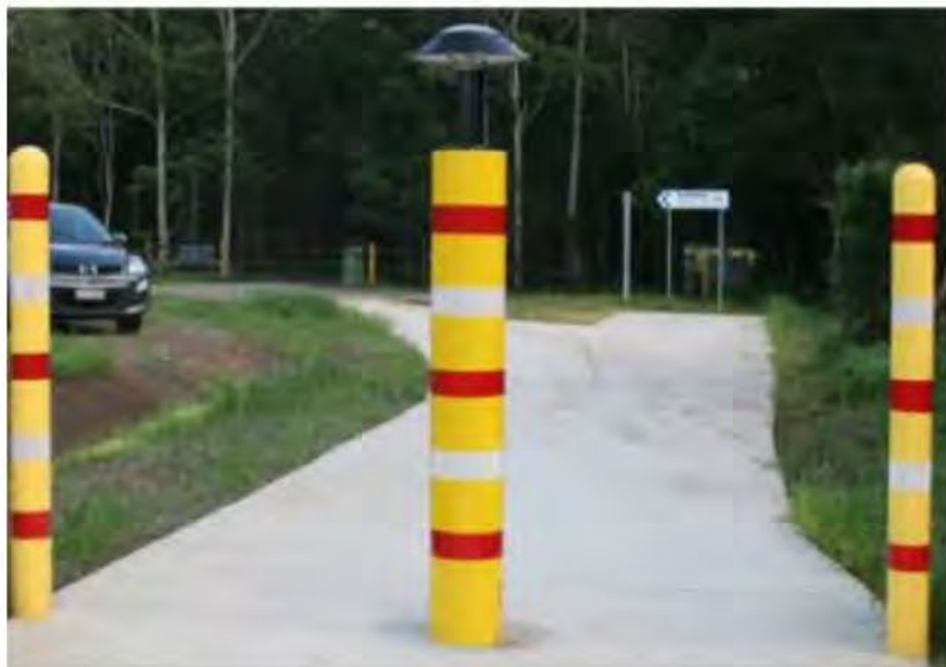
Figure 5-1: Bollard treatment at intersections
