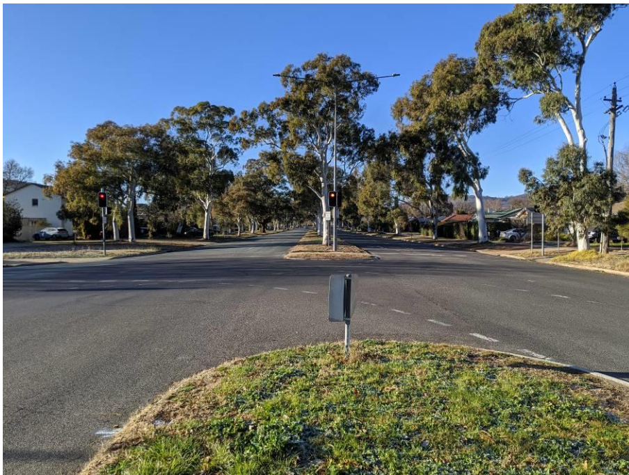
Photo 2-2 Phillip Avenue (southeast view north of the intersection with Windeyer Street)
