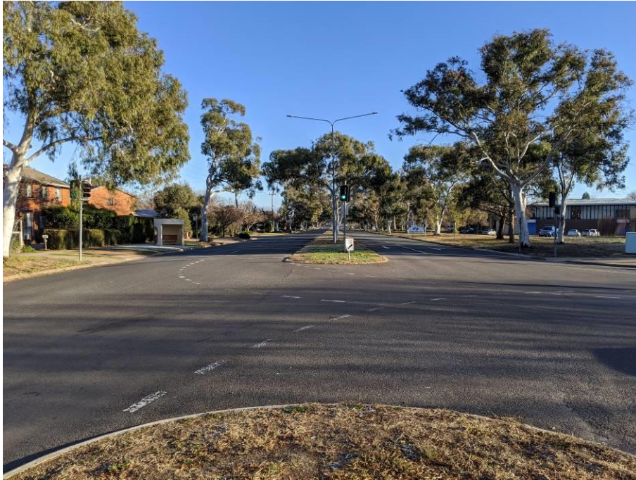
Photo 2-1 Phillip Avenue (northwest view south of the intersection with Windeyer Street)
