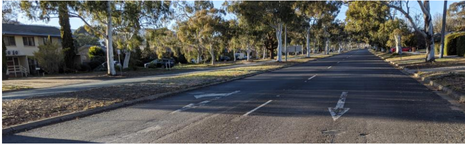
Photo 2-6 Existing pavement markings condition
