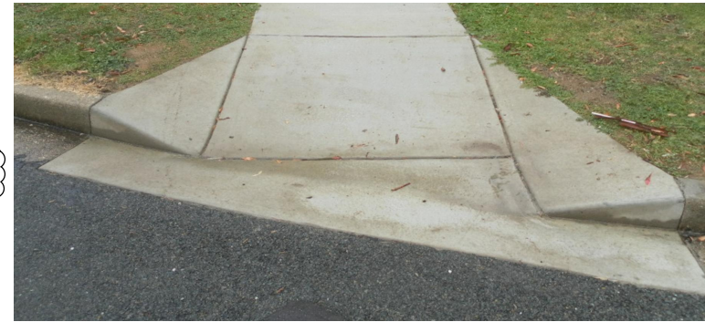
EXAMPLE OF SUBURBAN KERB RAMP
