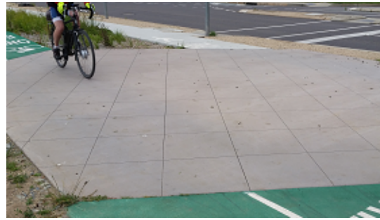
TYPICAL INTERACTION ZONE PAVEMENT WITH SAWCUT
