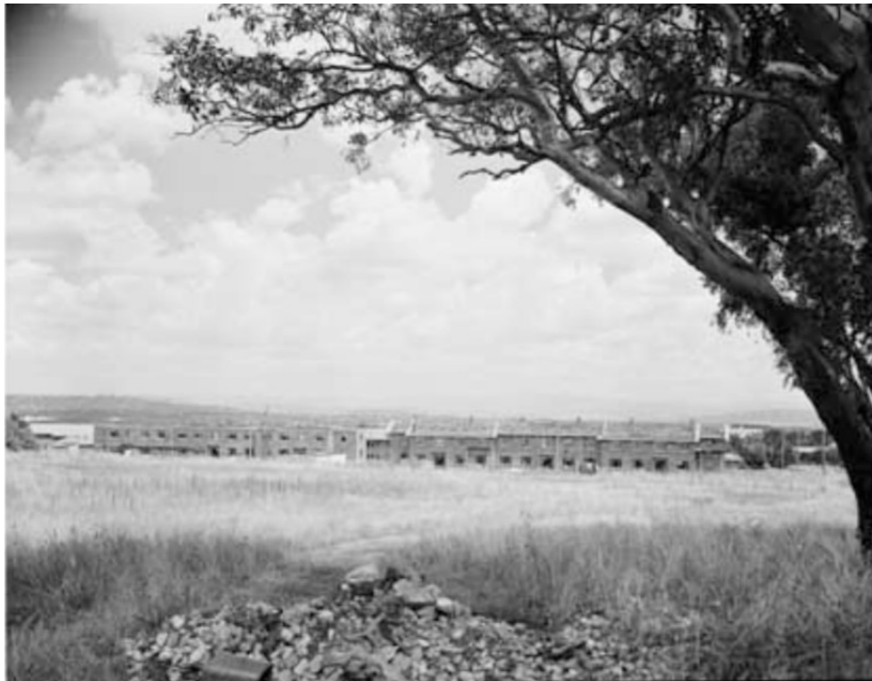
Figure 4: Ainslie Flats Under Construction 1951
