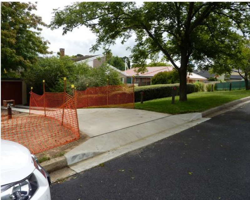
Figure 07- 2 Vehicle Crossing: between the road surface and the first expansion joint
