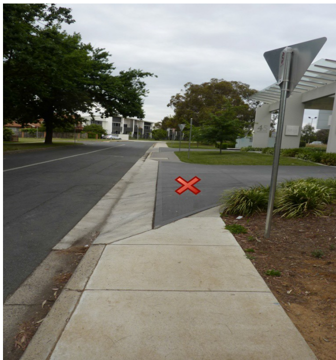
Figure 07- 4 Driveway with incorrect footpath priority
