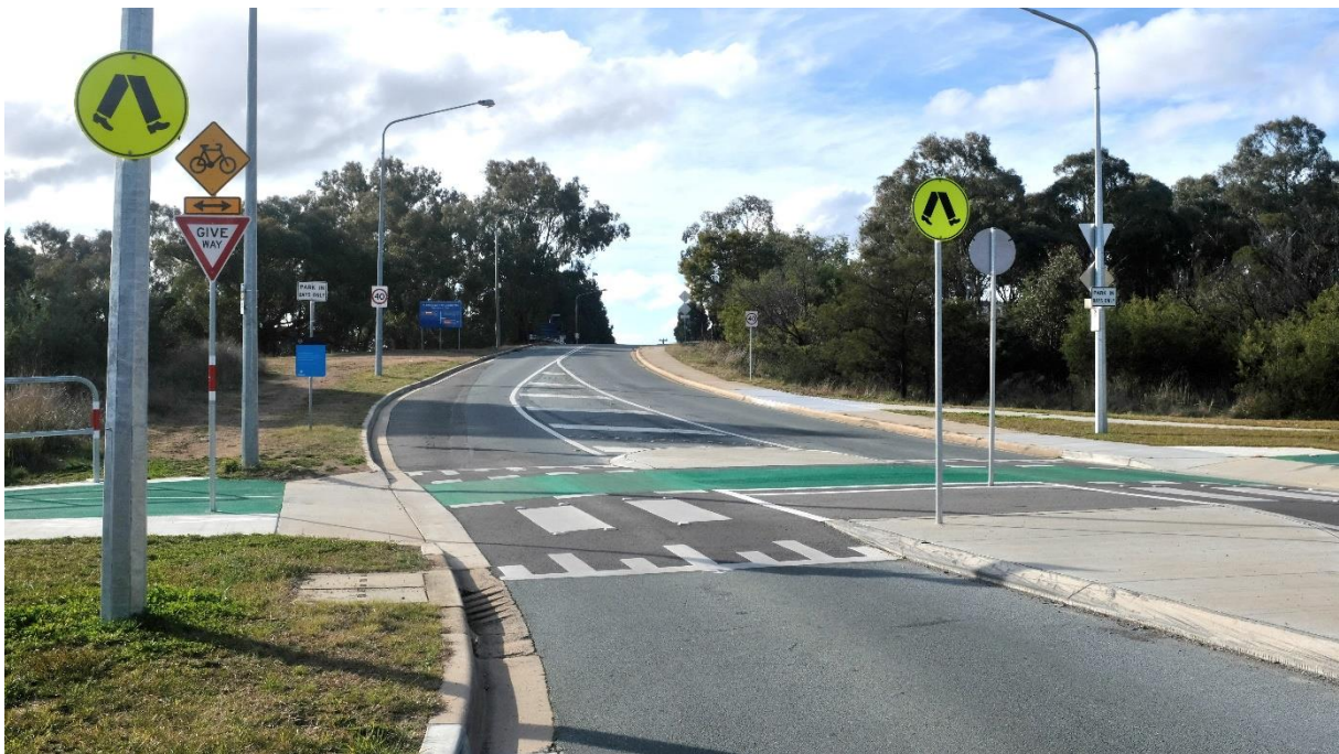
Figure 5-9 Bicycle-Only Priority Crossing adjacent Zebra Crossing on a local access street in Retrofit.
