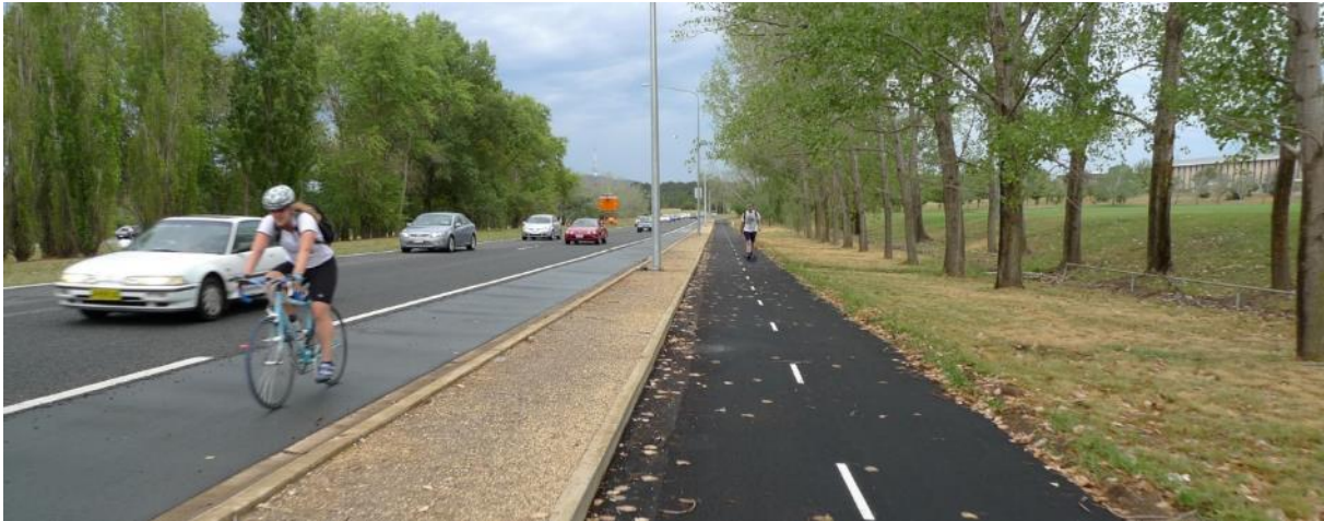
Figure 5- 13 Bicycle lane retrofitted to an arterial road. Bicycle lane on Adelaide Avenue divided carriageway at Curtin, ACT complemented by an adjacent trunk path serving both cyclists and pedestrians.
