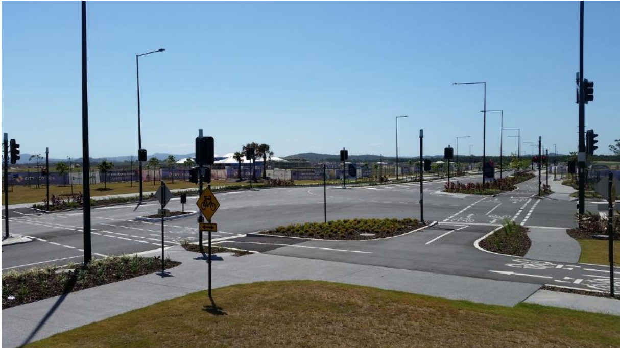
Figure 5- 10 Two-way bicycle-only paths at a signalised intersection.
