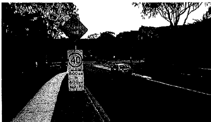
Photo 3-6 Palmer Street school speed zone sign
