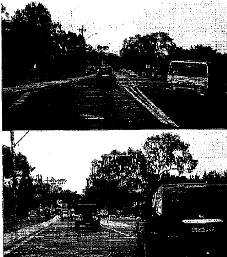
Photo 3-9 Visibility from drivers eye level (1.1 m) of the children's crossing for eastbound traffic
