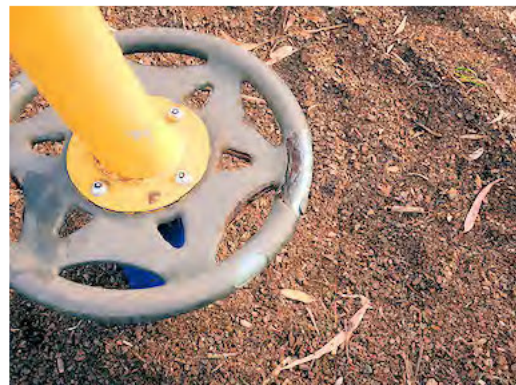
Photo taken: 08/04/2020 Rubber coating worn on foot pad. Monitor.
