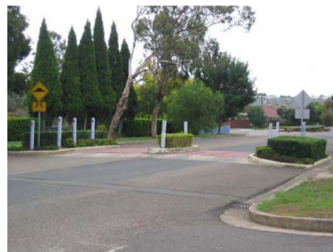
Raised platform – no pedestrian crossing
