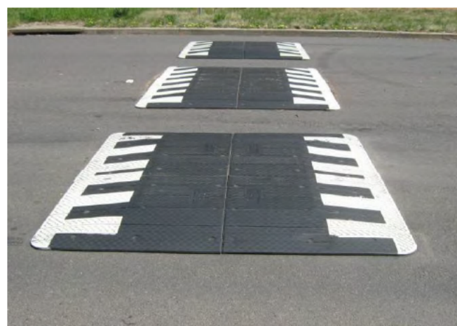
Speed cushions and prominent signage will assist in slowing traffic and improving safety on Coyne Street.
