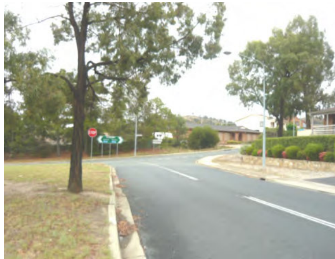
Coyne Street / Bugden Avenue intersection looking west
