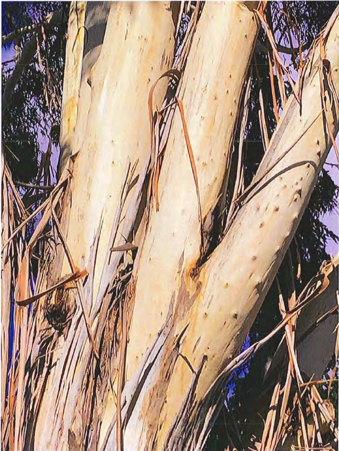
Figure 9: 'V' Section with Signs of Deterioration and Trapped Water (31 Jan 22)
