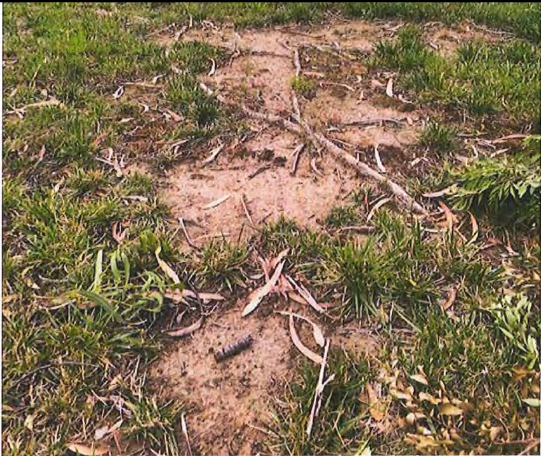
Figure 19: Encroaching Roots – Dead Lawn and Trip Hazards (12 Jan 22)
