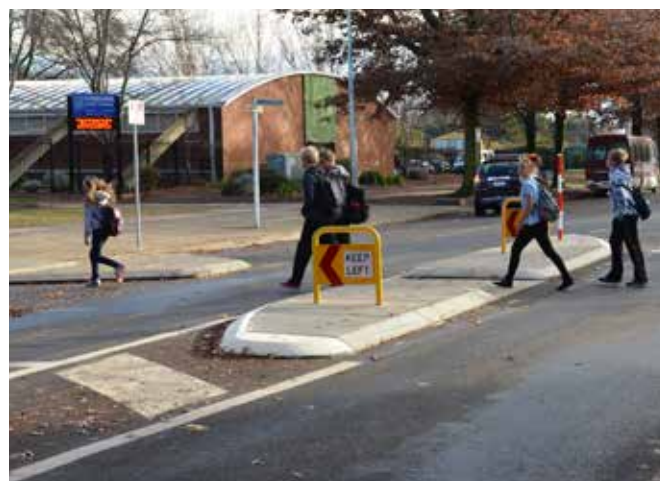
Photo 8: Refuge islands at Lyneham High School on Goodwin Street, Lyneham
