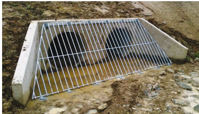
Figure 8-9 Typical culvert inlet protection grate
