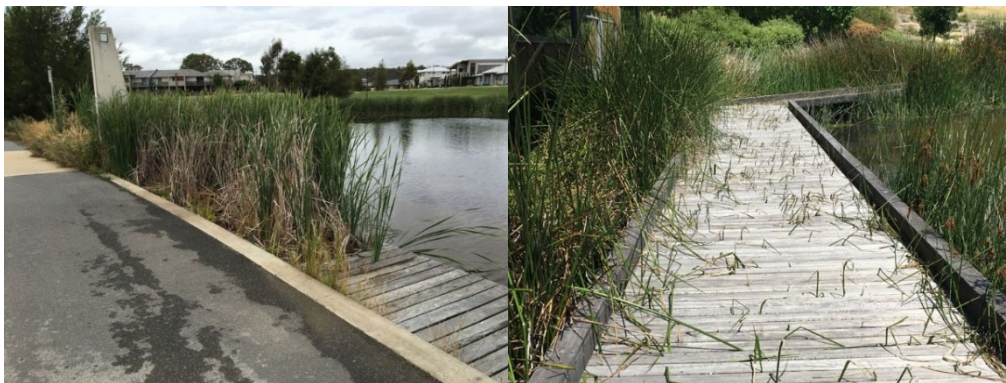
Figure 8-20 Typical examples of macrophyte growth through boardwalks
