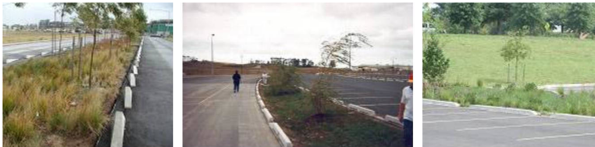
Figure 8-33 Bioretention swale kerb treatments
