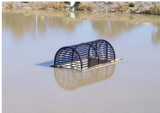
Figure 8-24 Typical primary outlet domed cover
