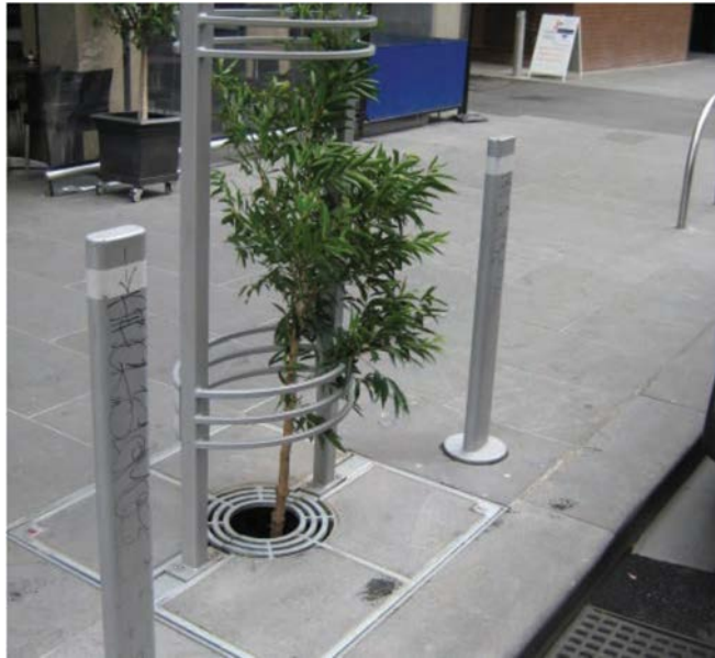
Figure 8-31 Example Tree Pit Cover (Melbourne Water)
