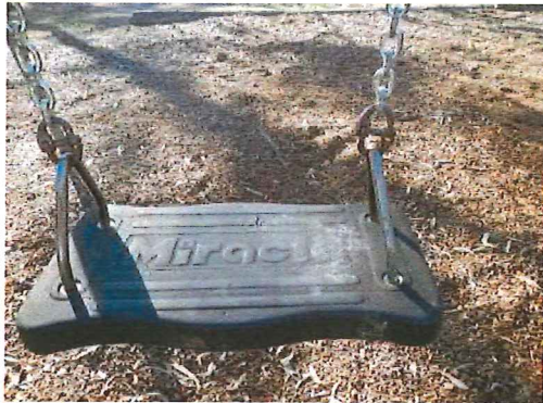
Photo taken: 24/05/2016 Bent suspension mounts.
