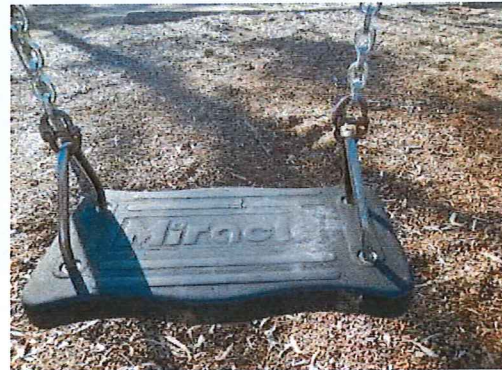
Photo taken: 24/05/2016 Bent suspension mounts.
