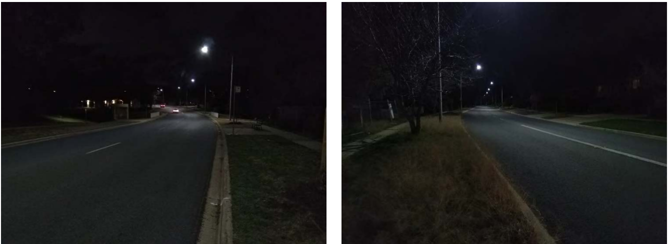
Figure 21 Street Lighting Conditions – Summerland Circuit
