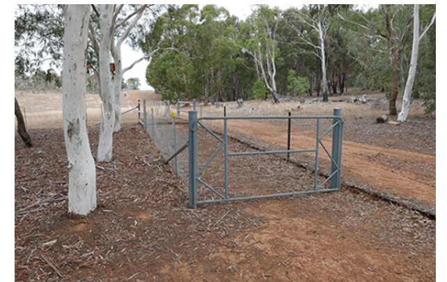
Constructed example with cavaletti step through horse gate and holding pen at corner of stock fences. North Lyneham.
